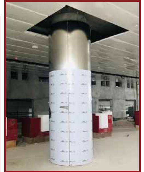
Revealing the stainless steel cladding
